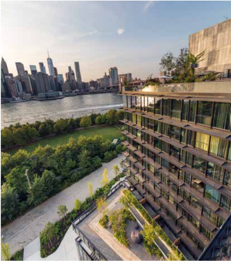
Pierhouse Brooklyn Bridge, NYC, USA
